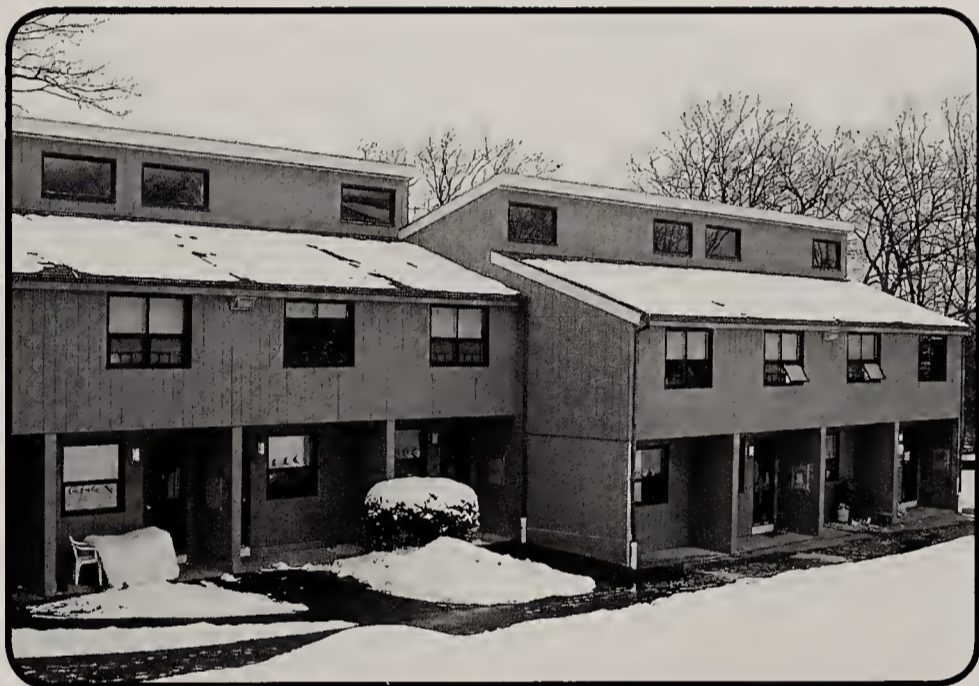
Bissonette Townhouses: The Bissonette townhouses are located behind Salisbury Hall in the "Hill" area of campus and are made up of 4-person apartments.
